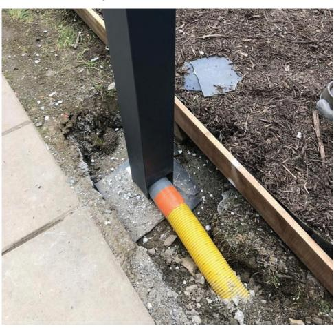
Otherwise the rainwater pipe can exit just above the ground level to drain away.
