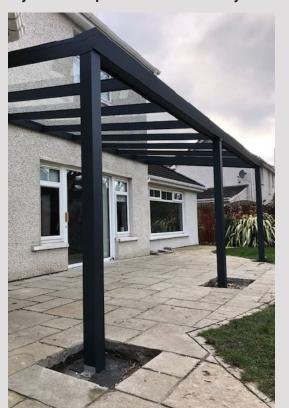
If you have a patio already installed then some sections will need to be lifted to allow for the concrete foundation pads to be installed, the paving can then be reinstated and cut around the veranda posts after the veranda has been installed. We can quote for this work locally or we can offer guidance and specifications if you wish to do this work yourself. Please note for Porcelain patios you will need your original contractor to carry out this work.
