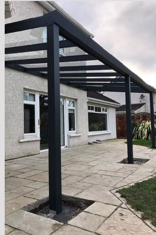
If you have a patio already installed then some sections will need to be lifted to allow for the concrete foundation pads to be installed, the paving can then be reinstated and cut around the veranda posts after the veranda has been installed. We can quote for this work locally or we can offer guidance and specifications if you wish to do this work yourself. Please note for Porcelain patios you will need your original contractor to carry out this work.
