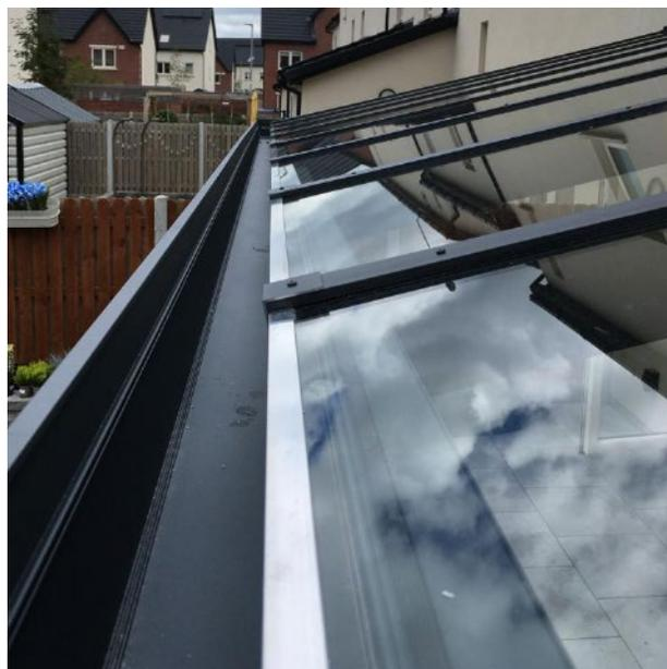
The Vesta Veranda has a choice of two gutter options, the Vesta and the Vesta Plus. Both options offer fully concealed gutters so no nasty gutter brackets, no sagging gutters. The downpipe is concealed within one of the upright posts and this can be connected underground to your existing
