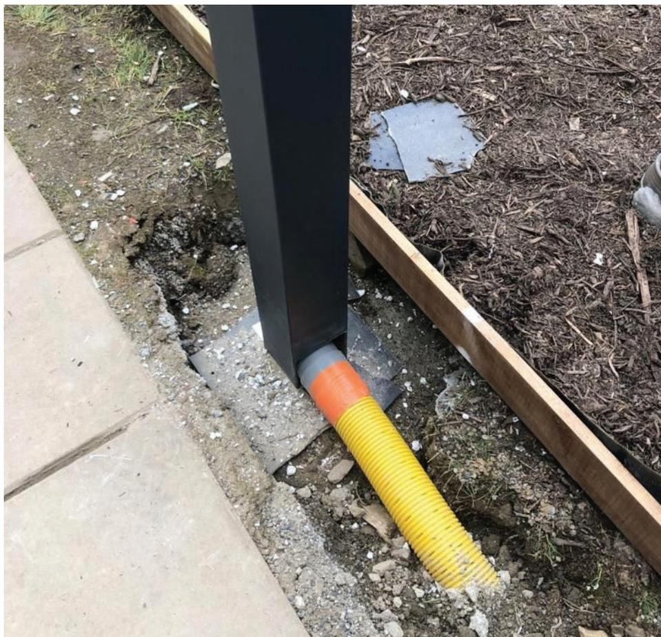
Otherwise the rainwater pipe can exit just above the ground level to drain away.
